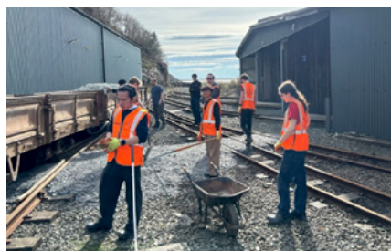
Preparing to ballast the far siding
