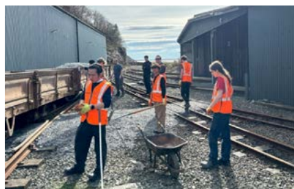
Preparing to ballast the far siding
