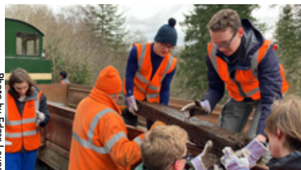
Lifting a sleeper up into the wagon
