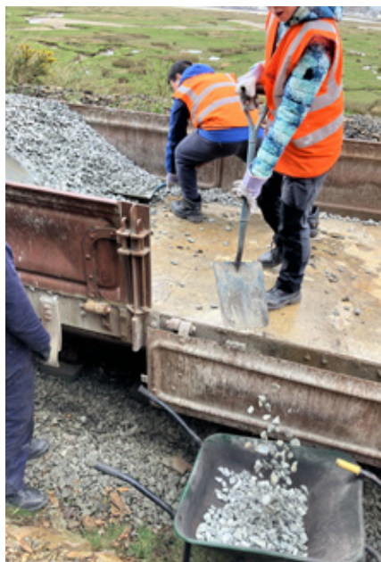
Ballasting the tracks
