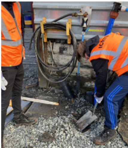
Digging gravel around a pipe
